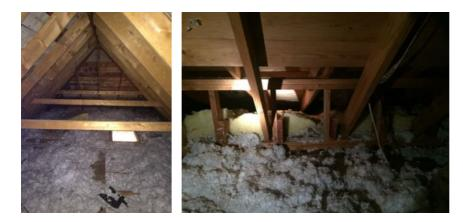
**Roof Framing Type** Wood Trusses, Joist and Rafters Condition: Satisfactory
